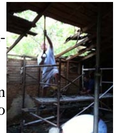
BK Stan Williamson knocks out the old roof of the garage.
